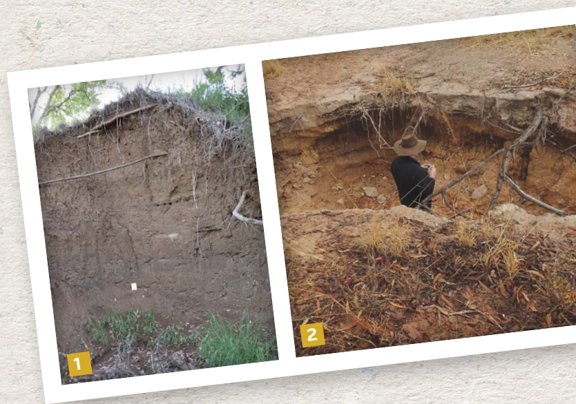
Photo 1: A 4.5m tall eroded bank created after an intense storm
