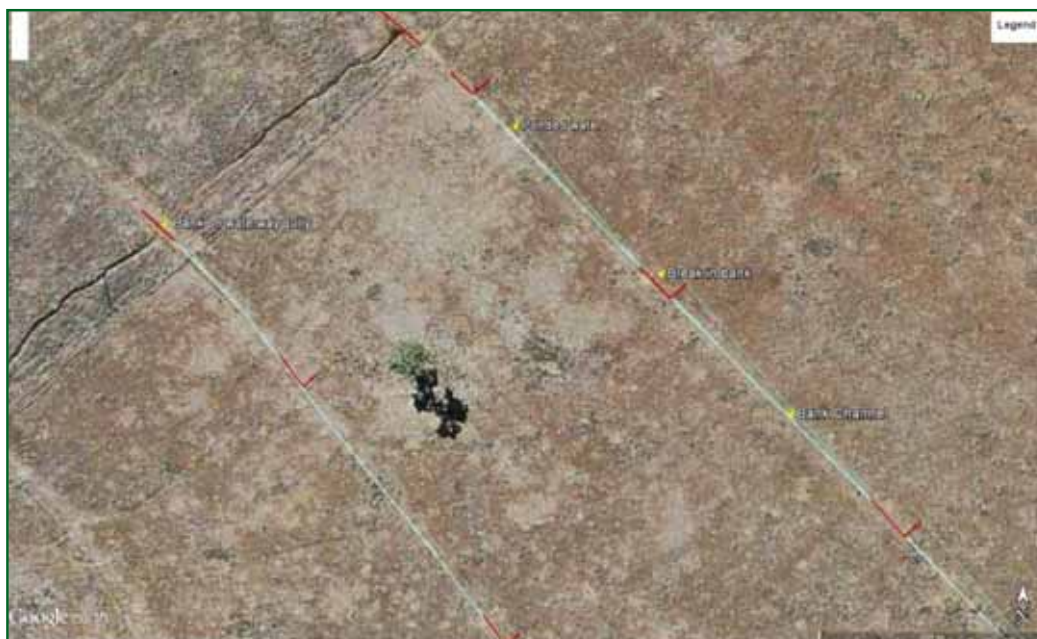
FIGURE 2: Close-up of breaks and expected pondage design
