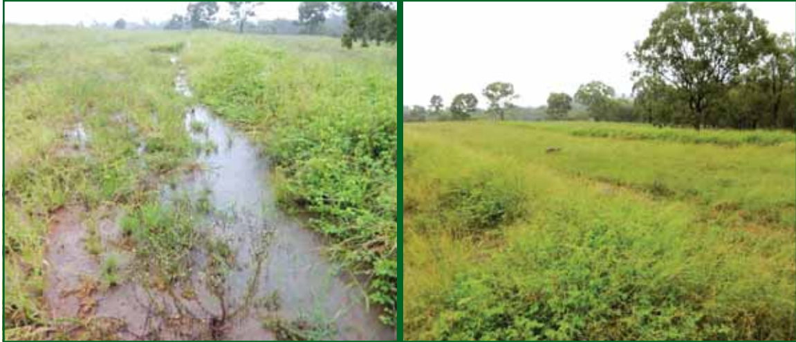
PHOTO 6 & 7 : The Site / After Construction and Heavy Rain
