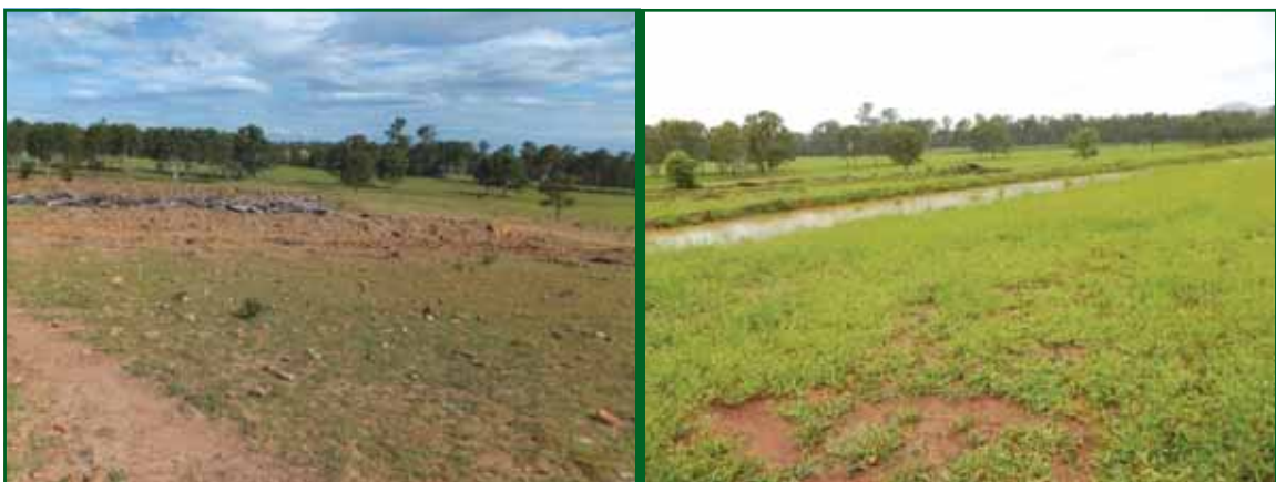
PHOTO 4 & 5: The Site / Before and After Construction
