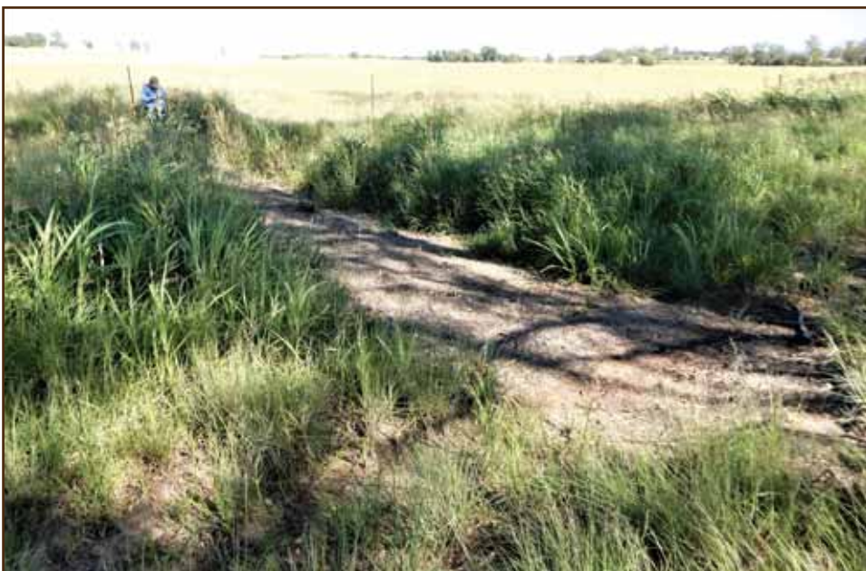
SITE 1 PHOTO 70: Grassed waterway post-construction of the weirs, after good rain.
