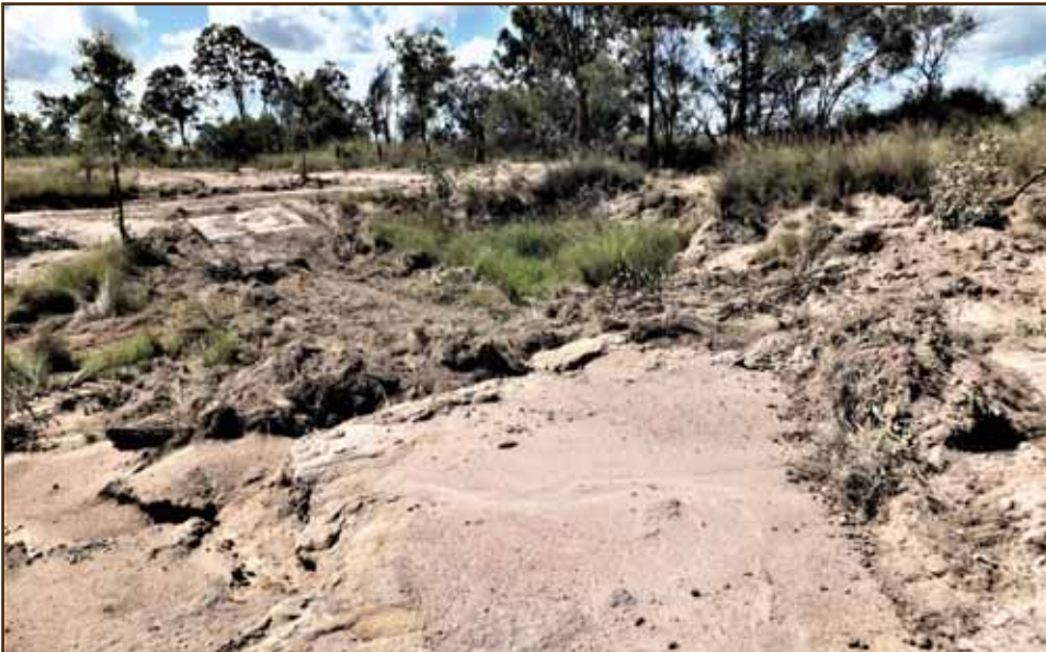
PHOTO 39: Rock chute site after initial site preparation.
